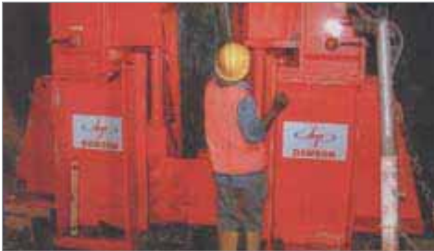
The X-400 working underground Marina Square, Singapore extracting H-Pile
