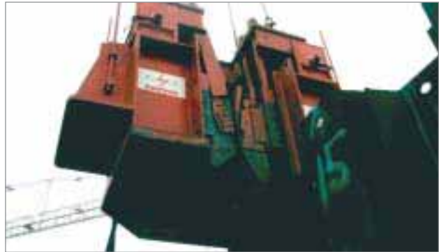
The X-400 at London Heathrow Airport extracting Sheet Pile
